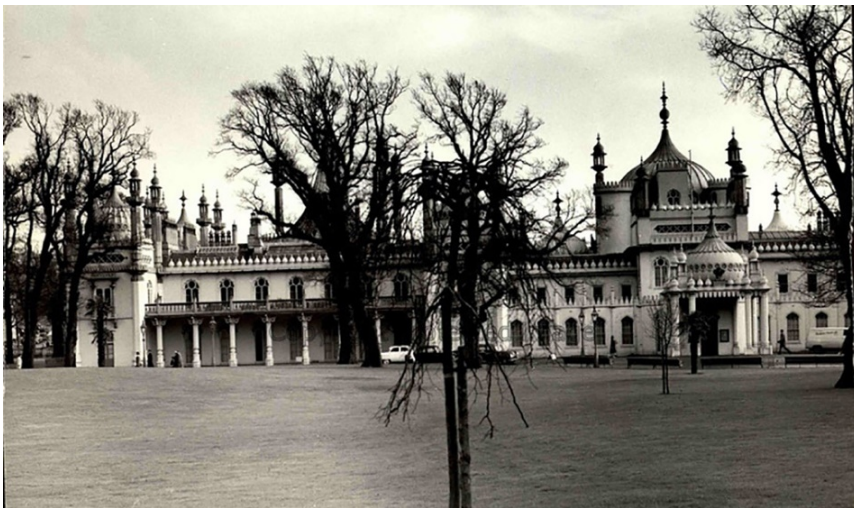
1960s photograph of west front showing mature elms along north-south drive, shortly before their loss to DED and later the 1987 storm (courtesy Peter Bourne)
