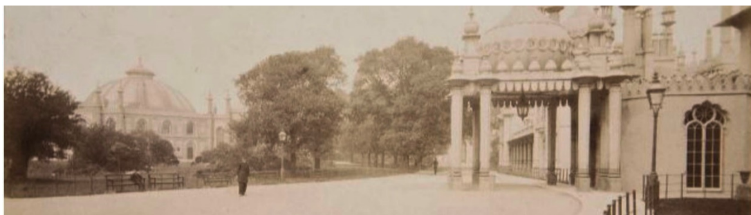
View 1 looking north 1870s showing rows of mature elms lining drive (Regency Society)
