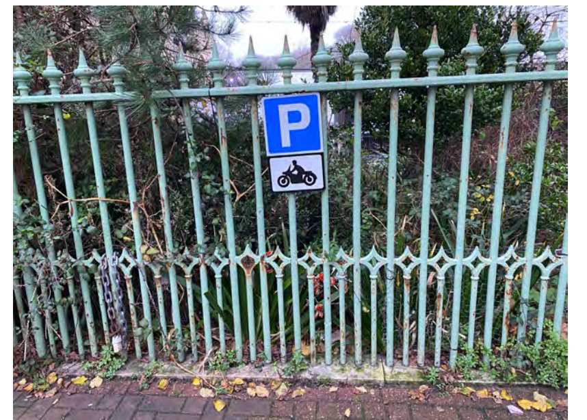
Existing Palace Place railings
